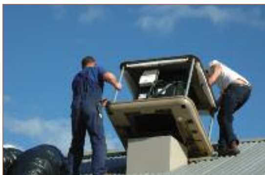
Maintenance of air-conditioning system
