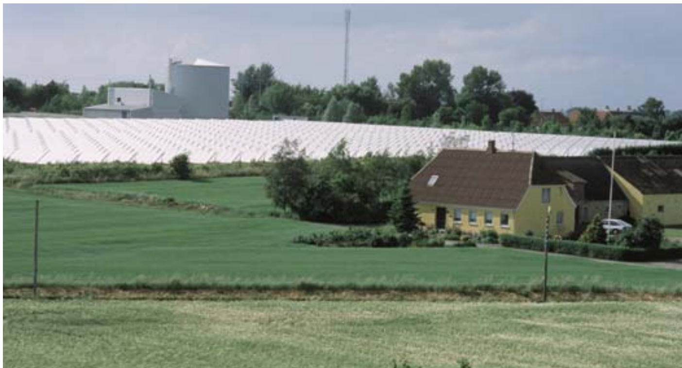
'Solar park' at Marstal (Denmark).
