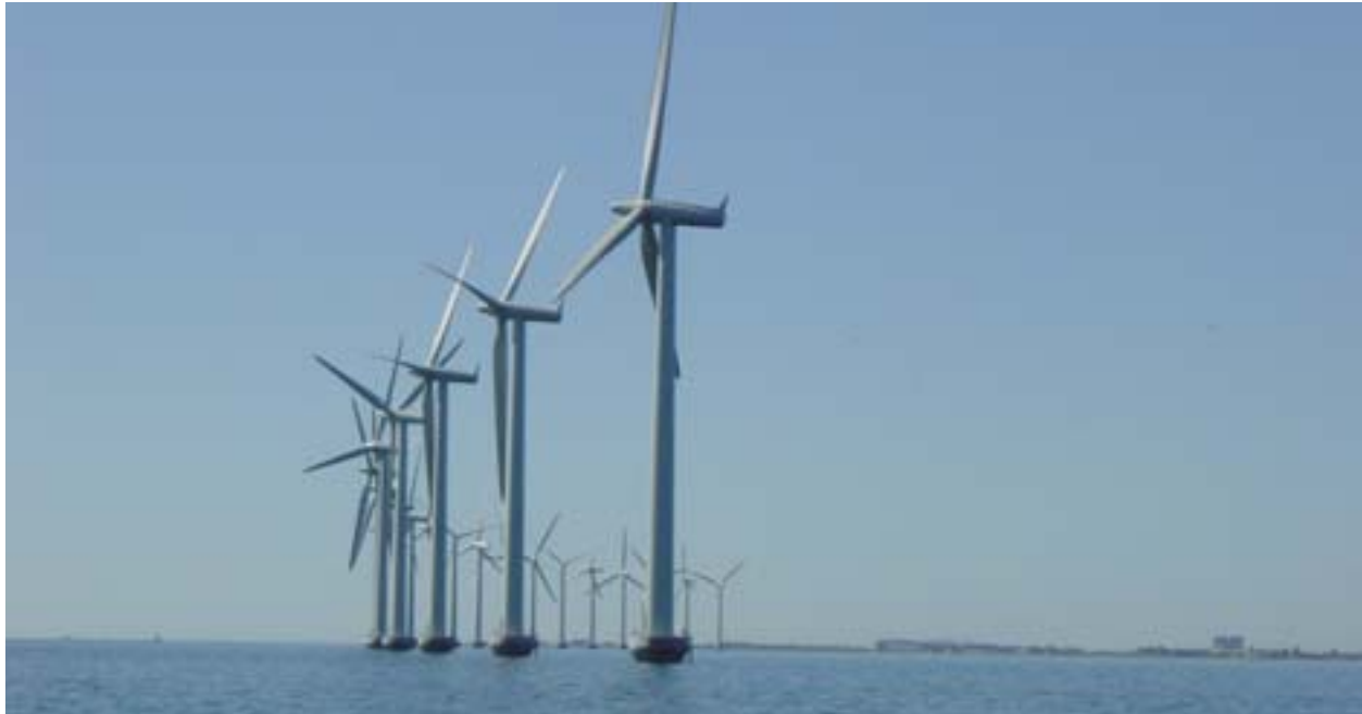
Offshore windfarm near Copenhagen (Denmark).
