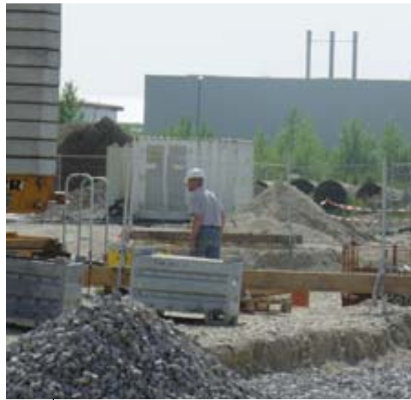
Construction of a biodiesel refinery at Enns.
