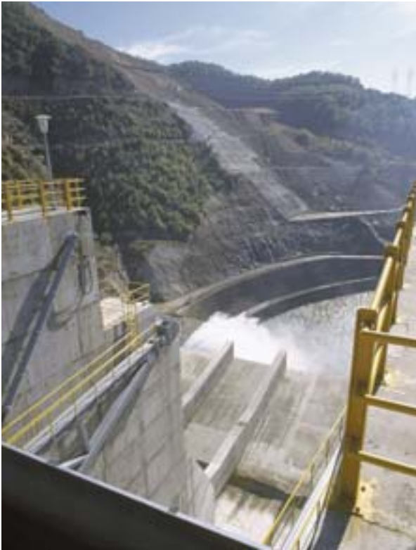
Hydroelectricity without borders: dam on the Nestos river, between Greece and Bulgaria.
