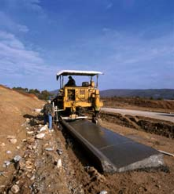
Construction of a new road between Greece and Bulgaria.
