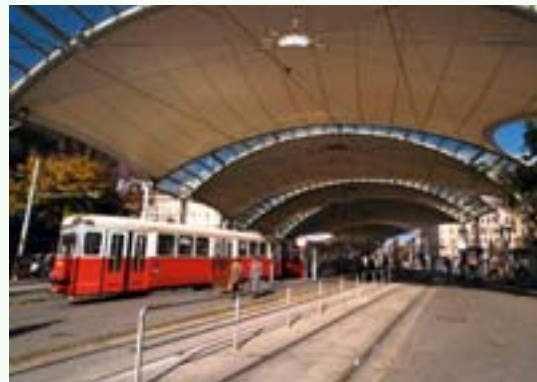
URBAN renovation in Vienna, Austria.
