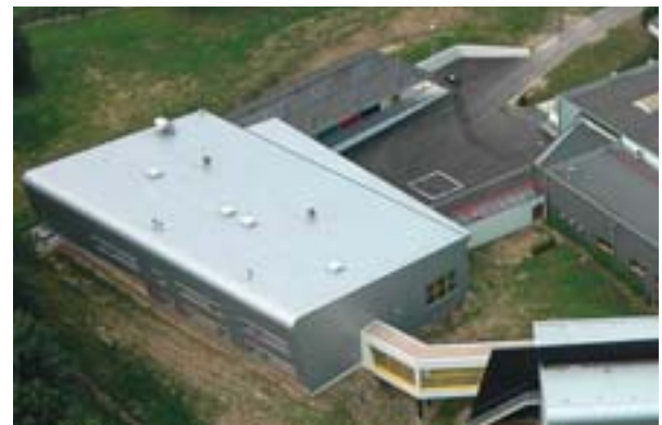
The Regional Centre of Innovation and Technology Transfer (CRITT) at Charleville-Mézières, France.
