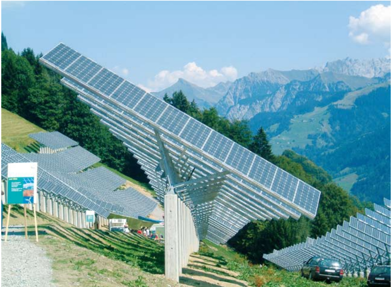
A large photovoltaic system produces 530 MWh from solar energy in Blons, Austria.
