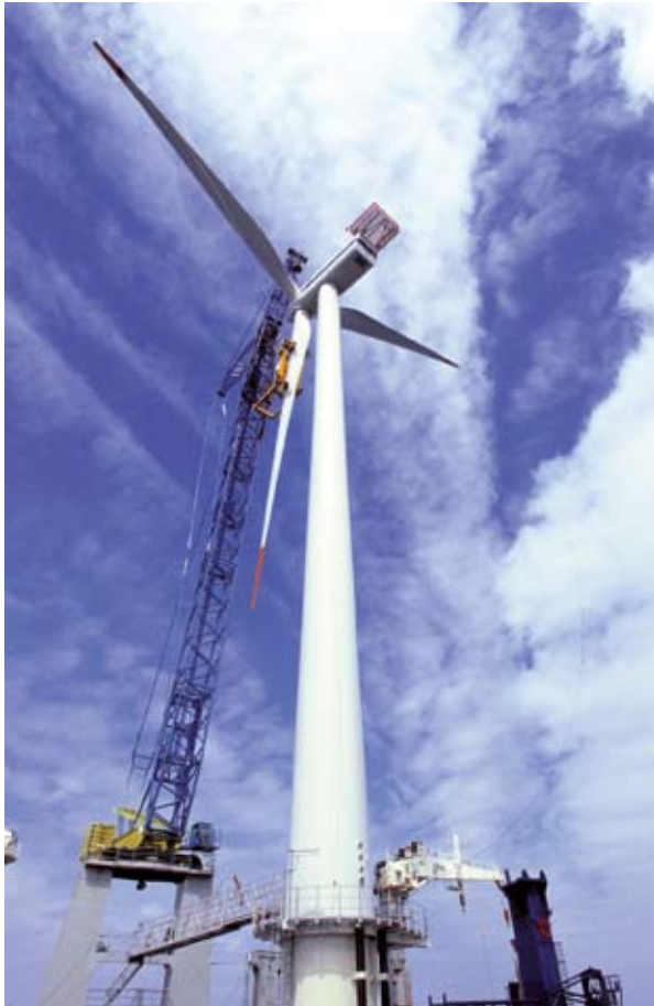
Setting up an offshore wind turbine.
