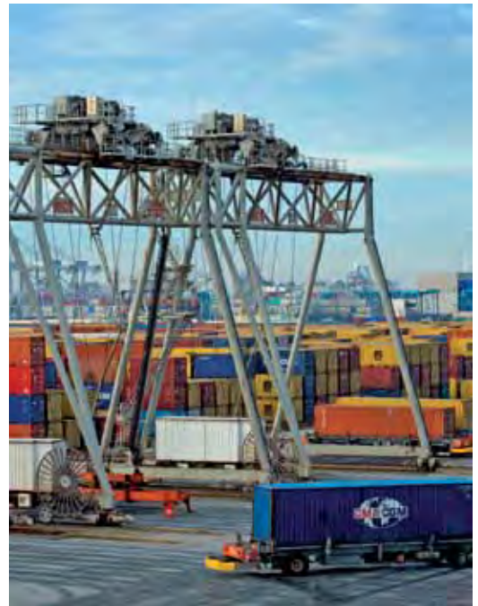
Connecting Europe facility — Europe Container Terminals (ECT) in Rotterdam, Netherlands.
