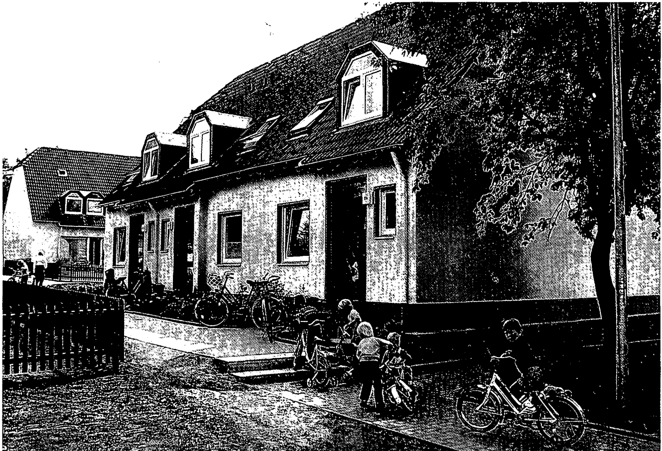
Construction of workers' housing — Glückauf Dh — Homberg
