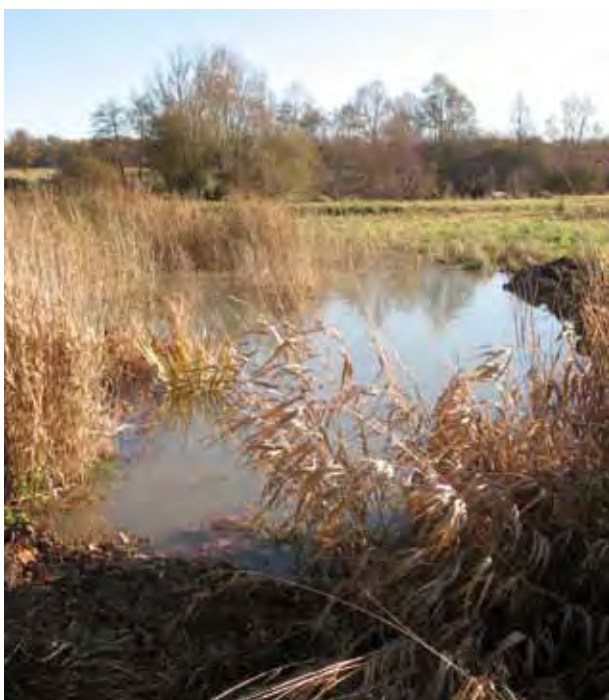
The artificial wetland and the parallel arterial ditch stored and degraded most pesticide fluxes
