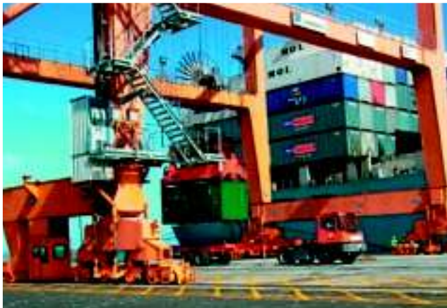
Mauritius Container Terminal II project, signed in 2004 (own resources).
