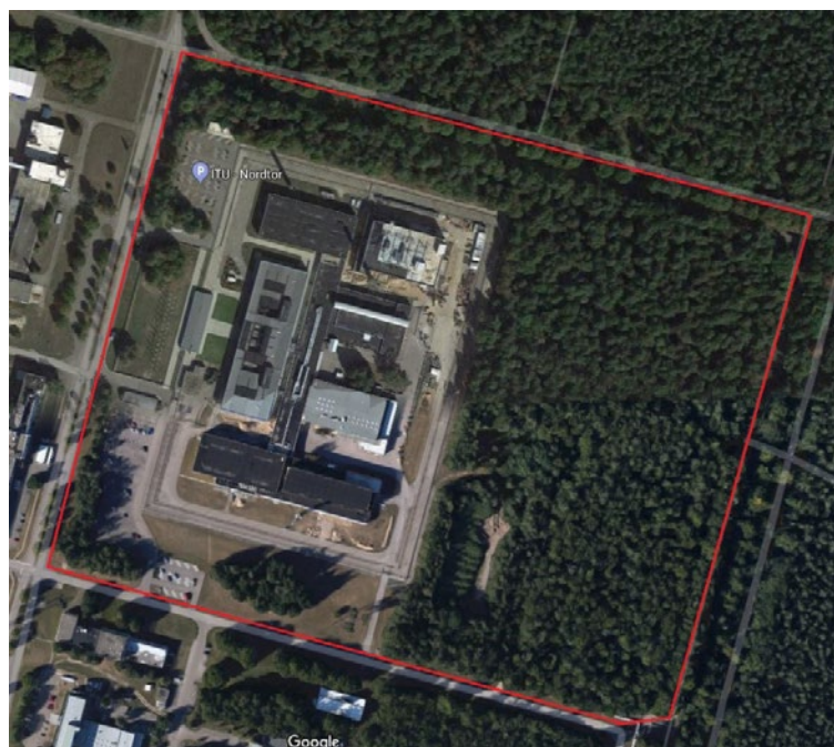
Figure F18: Aerial view of the site including “natural” parts
