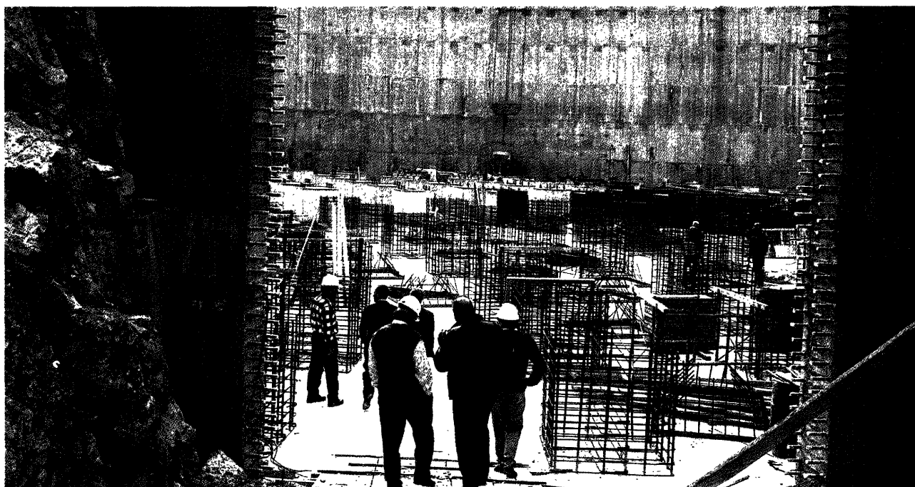
Liquefied natural gas tank — DEPA, Greece
