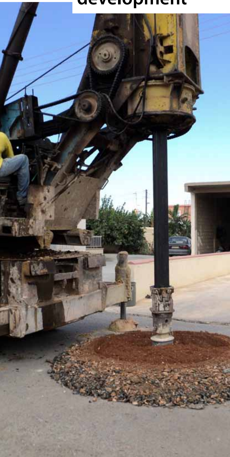
Manhole drilling
