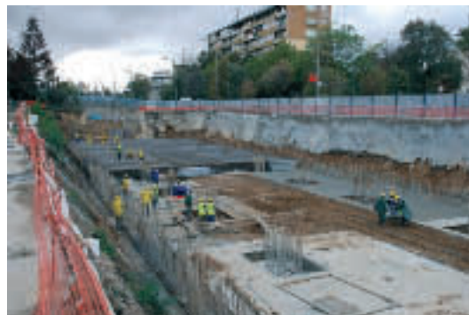
Station construction – Aug 2009
