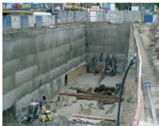
Tunnel construction – Aug 2009
