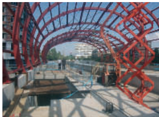
Construction of metro station
