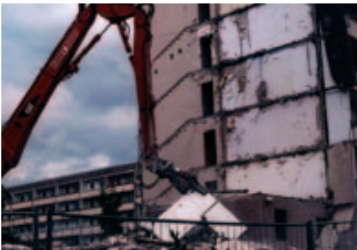
Cautious removal with a gripper-like demolition tool
