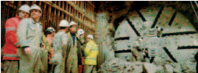
The tunnel-boring machine
