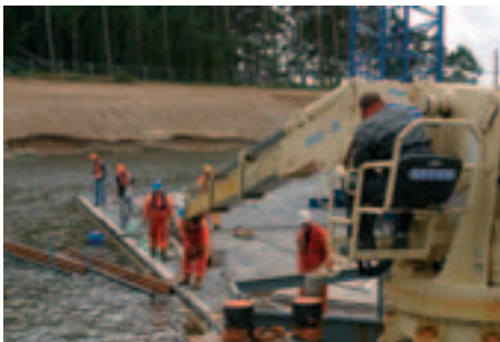
Immersion of the tunnel elements (courtesy of Heinrich Hirdes GmbH)
