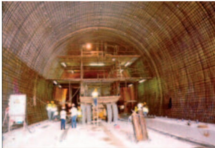
The tunnel in Dodoni Reinforcement positioning in tunnel
