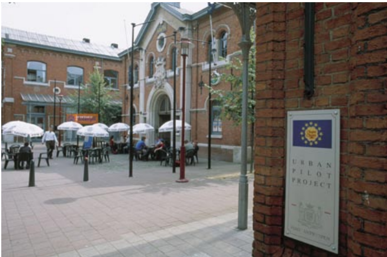
The NOA centre in Antwerp, Belgium, provides services for 15 small businesses and a local café for the neighbourhood.
