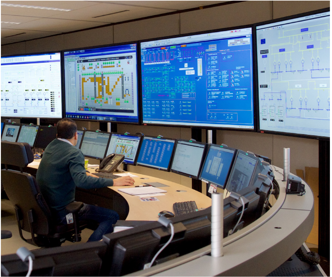
Control centre of the centralised technical management system of the Justus Lipsius building
