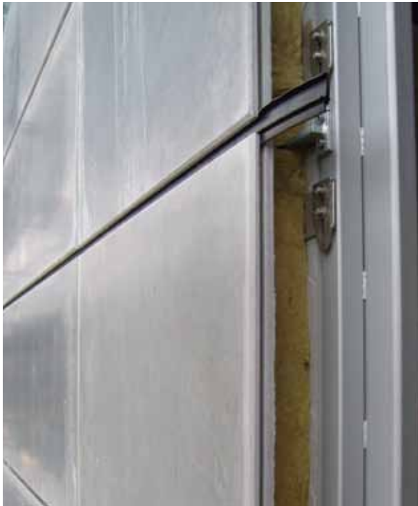
The basic element of construction is made of two shells of textile reinforced concrete combined with rigid polyurethane foam insulation
